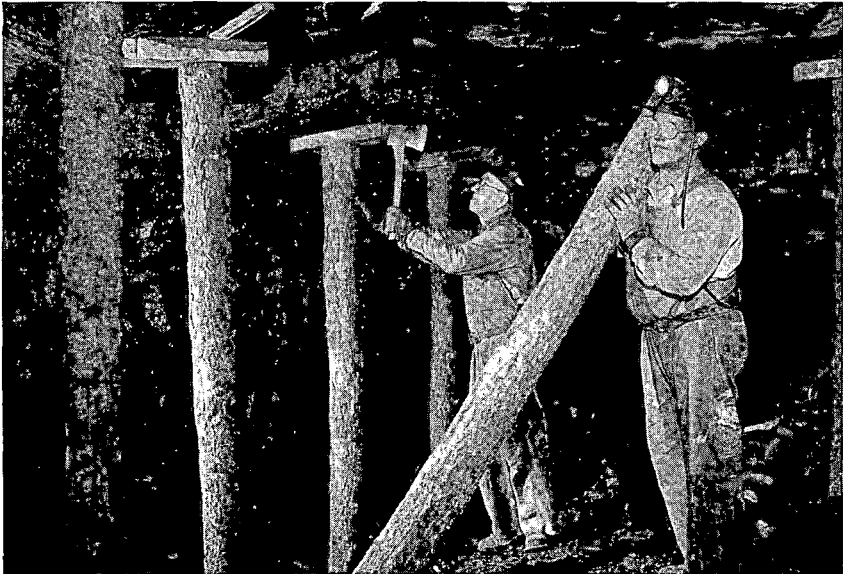
With hardhats and electric lamps, which had long since replaced caps and open-flame lamps, miners set timbers at the Colorado Fuel and Iron Company's Morely Mine in 1956. Photo courtesy of CF&I Steel Corporation.
